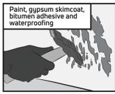
Chip surface (min 80%). Remove bitumen adhesives and waterproofing completely. Apply a TAL Keymix & TAL Keycoat primer slurry.
