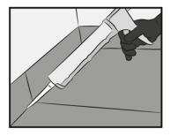
Construct tile panel movement joints – soft joints – located at max 5m centres for interior surface bed and wall applications, and max 3m centres for suspended applications and exterior applications, as well as around the perimeter of all floors and in all vertical corners. Joints must be minimum 5mm wide and extend through the tile and tile adhesive layers. Fill joints with **TAL Goldstar Sealmaster 1000** polyurethane joint sealer.
